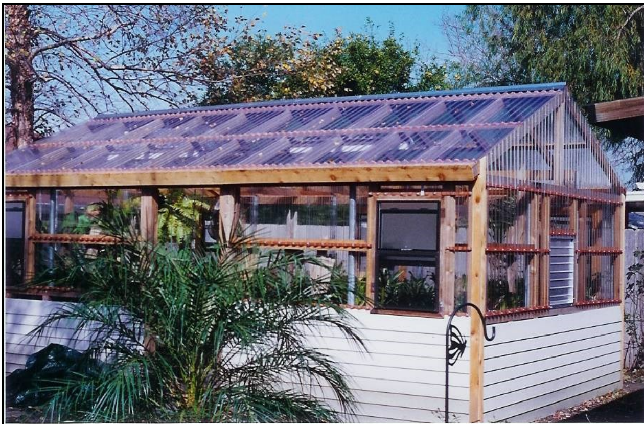
I built my greenhouse 20 ft. x 12 ft. with 7 ft. walls
